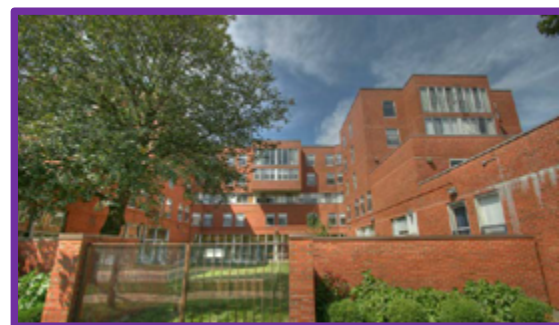
1) Renovation of New House (W70) began in 2017.
