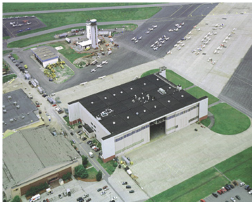
Hanscom Field Flight and Antenna Test Facility
